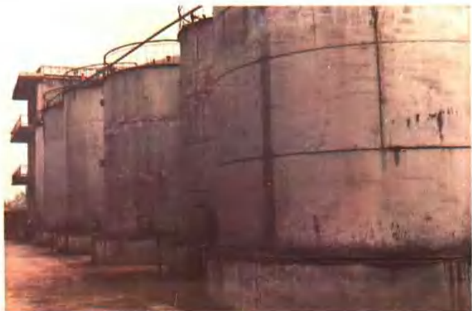
团风油厂油罐
